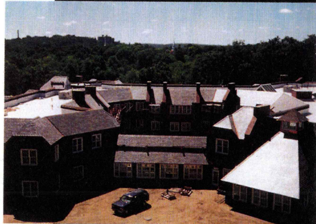
Slate & copper cornice work Carmel Terrace, Framingham, MA
